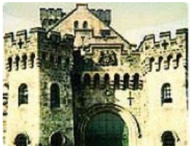
Armley Gaol, Leeds. Built 1847.
