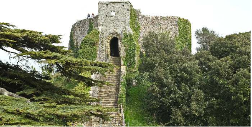
Fig. 1. Carisbrooke Castle shell-keep, c. 1130-40 with added gatehouse and portcullis c. 1335.
