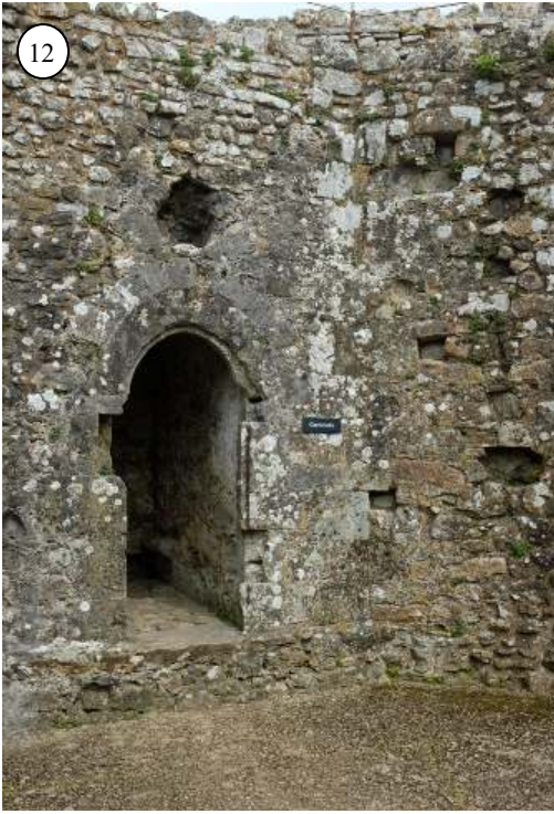
Figs. 12-15. The interior of the shell-keep. 12: Garderobe (inserted early 14th century?) on the east wall (with no dogleg). 13: Garderobe on the north wall (also seen in fig. 14, right). 14: Looking west along the curious high-walled corridor to the entrance gatehouse. Probably a post-medieval 16 th -century addition. 15: One of two arrow loops on the top of the gatehouse.
