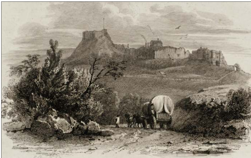
ABOVE: Fig. 2. After Luke Clennell (1781–1840) 'Carisbrooke Castle from the Calbourn Road' From 'Picturesque Views on the Southern Coast of England', 1814.
