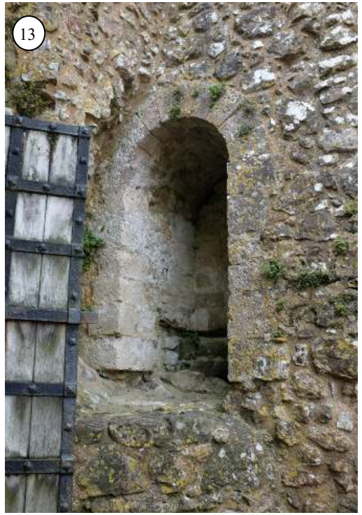
Figs. 12-15. The interior of the shell-keep. 12: Garderobe (inserted early 14th century?) on the east wall (with no dogleg). 13: Garderobe on the north wall (also seen in fig. 14, right). 14: Looking west along the curious high-walled corridor to the entrance gatehouse. Probably a post-medieval 16 th -century addition. 15: One of two arrow loops on the top of the gatehouse.
